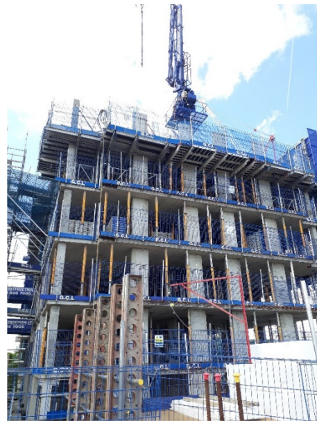
Figure 6.2 – Example of In-situ Flat Slab Construction
