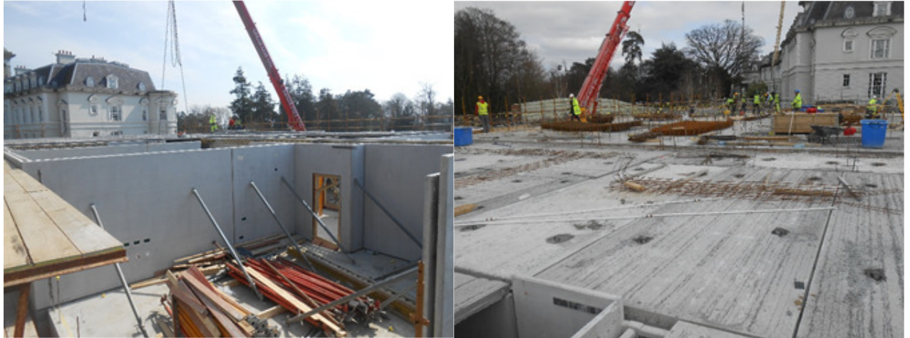
Figure 6.3 – Precast Concrete Frame Construction
